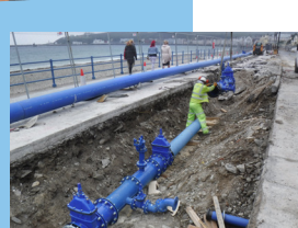
New utility infrastructure has been installed
